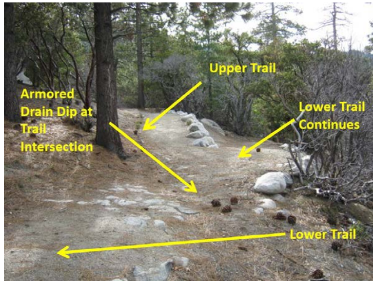
Photo 12.4 - Trail Intersection with Armored Drain Dip
