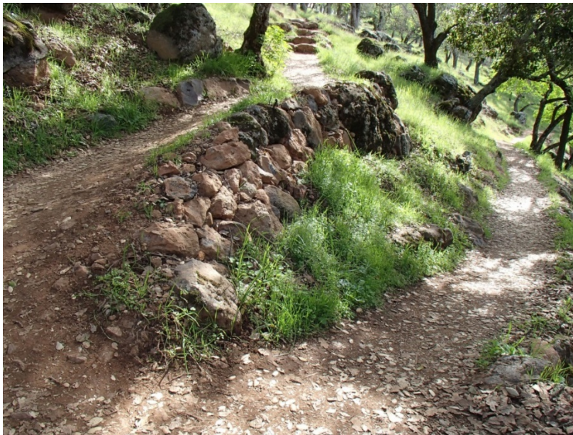
Photo 12.2 - Use of Barriers Between Legs of a Switchback
